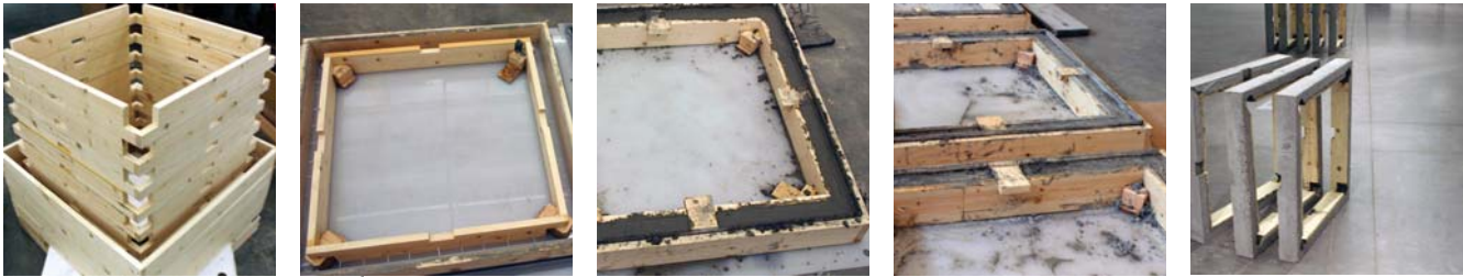
constructing concrete frames
